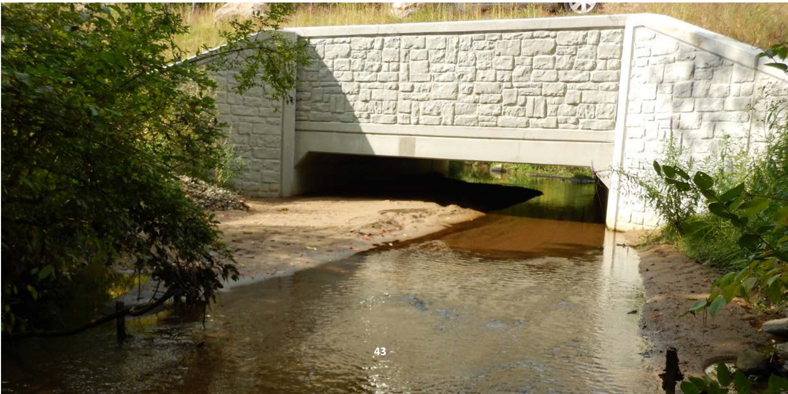
Open-bottom box culvert at McQuesten Brook and Eastman Ave., Bedford, NH – credit: Melinda Bubier
