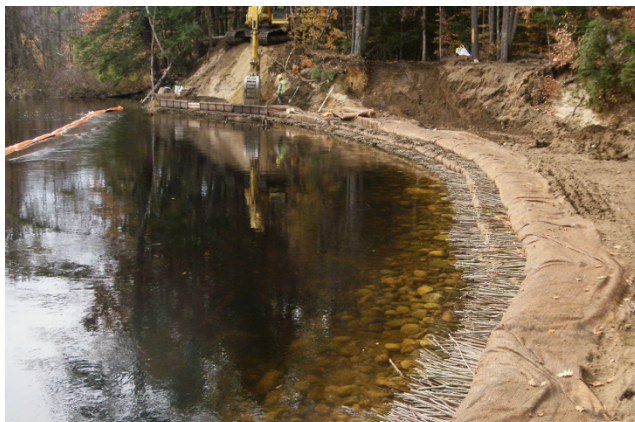
Streambank stabilization with brush layering during and post project – credit: Craig Rennie
