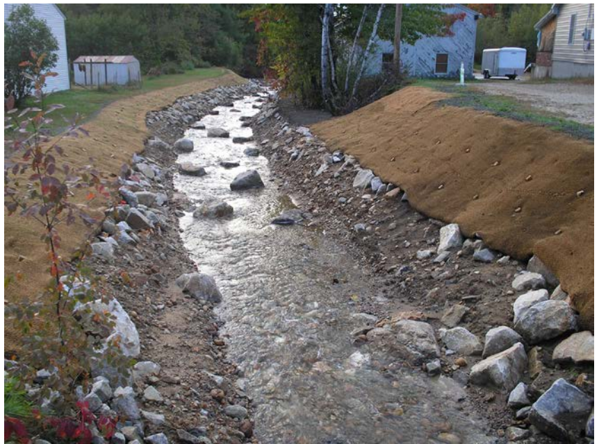
Leighton Brook bank stabilization, Epsom, NH – credit: NHDES Staff
