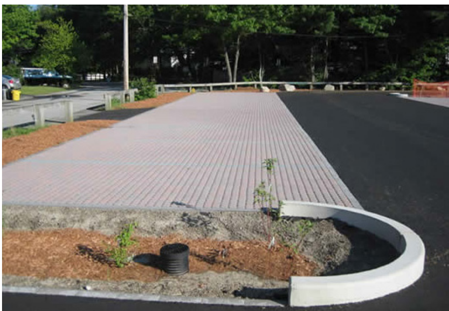
Pervious paving and bioretention in a parking lot – credit: Mass.gov
